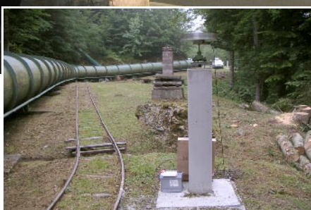
Topometric monitoring of the pressure conduit of Le Bious (Pyrénées-Atlantiques)
