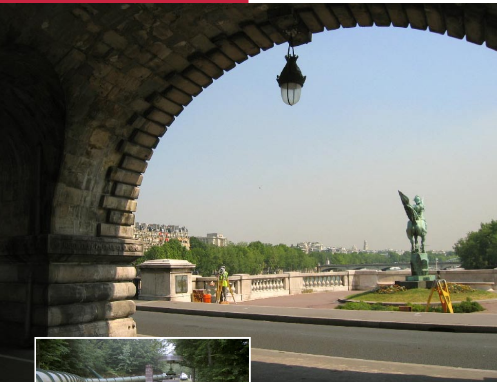
Topometric monitoring of the Viaduct of Passy (Paris)
